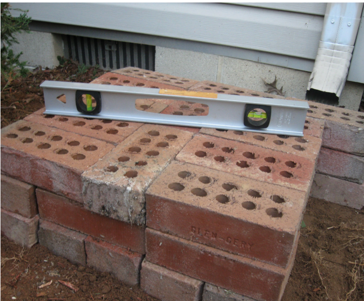
Figure 2. Brick platform used to elevate a rain barrel. The ground below the platform should be leveled out before installing a rain barrel.
