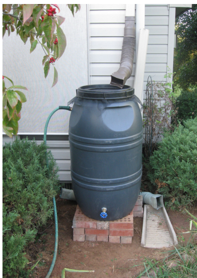
Figure 1. Fifty-five gallon rain barrel made from a recycled olive barrel. A plastic downspout extension is used to direct water into the barrel.
